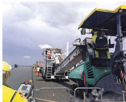
Using the material transfer vehicle helped reduce thermal segregation
