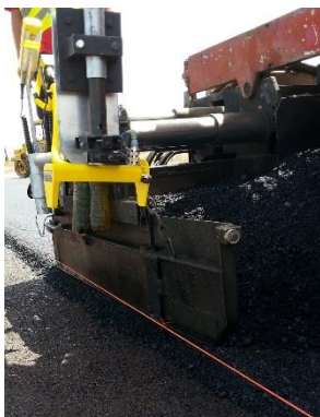
The Sonic-Ski plus ultrasonic sensor can use both a cable or the substrate as a reference
