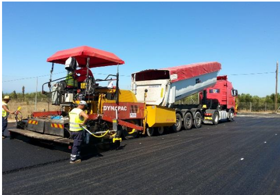
Test track construction in Greece with the MOBA-matic II levelling system
