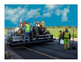
The temperature scanner measures the temperature of the asphalt over a width of up to eight meters depending on the measurement angle and mounting height
